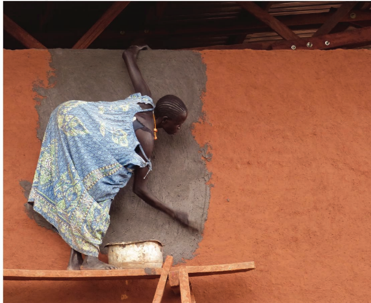
← Testing of prototype with local force Last coat of outside plastering in traditional technique →
