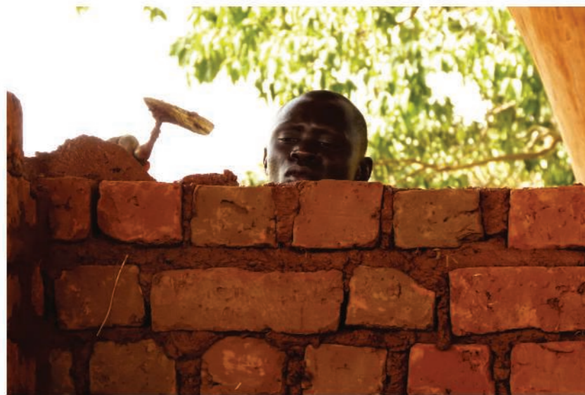
← Mason, building up an Adobe-wall
