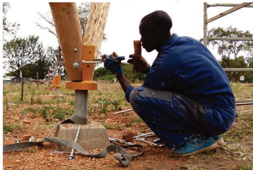
Carpenter working on termite-shield →
